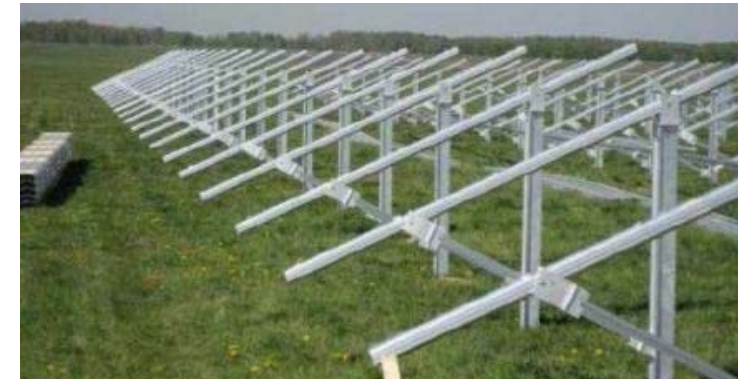
Photo 1 : Structures de support sans modules
